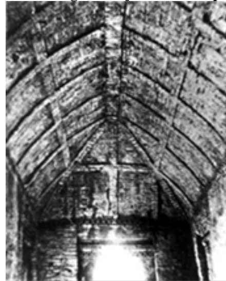
Figure 9: Chauchala vault in terracotta brick design, Masjidbari Mosque
