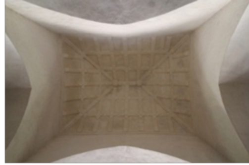
Figure 7: Chauchala vault of Sixty Dome Mosque, Bagerhat
