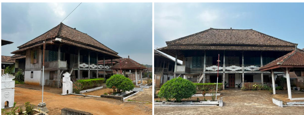
Figure 4. Building case study. (facing South)
