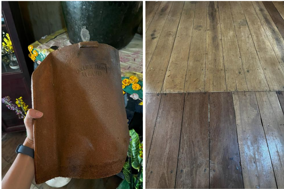
Figure 5. Roof (left) and floor (right) covering materials.
